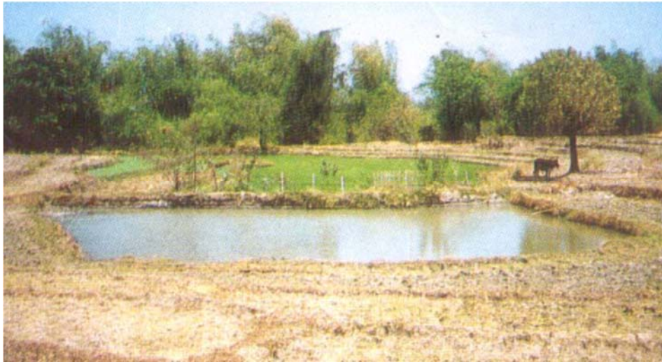
Micro reservoir “Small Farm Reservoir (SFR)”
